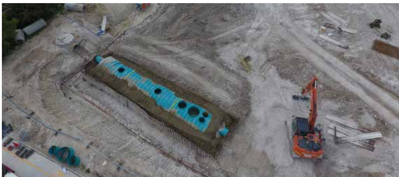
SPEL system installation. Yard extension, Soham, UK.
