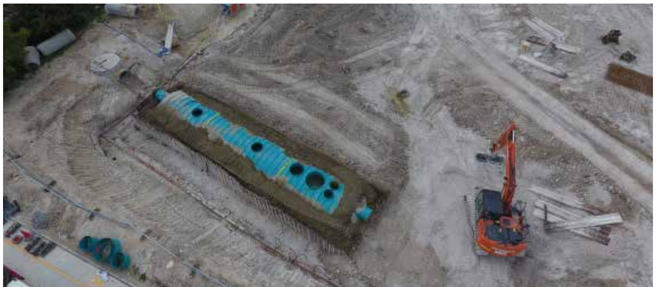
SPEL system installation. Yard extension, Soham, UK.
