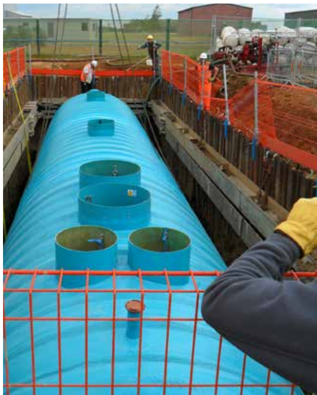
Dewatering at RAF Coningsby
