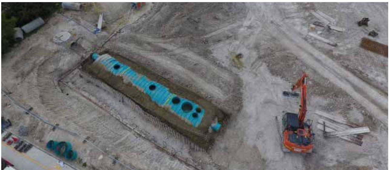
SPEL system installation. Yard extension, Soham, UK.
