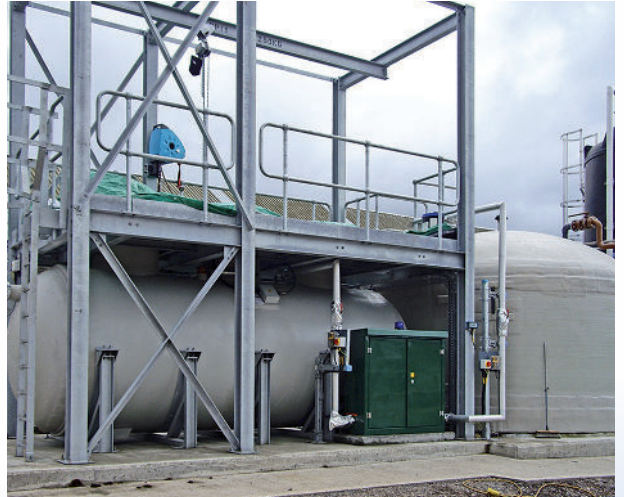
SPEL Separators are also designed and manufactured for above ground installations. The separator can incorporate secondary containment (bund), galvanised access platform and servicing equipment.
