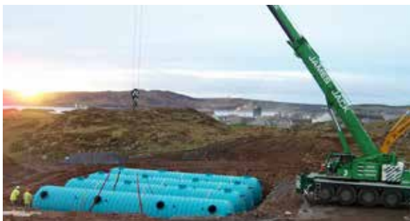
SPEL Septic Tanks 600 Series 240,000 litre Port Ellen, Islay, Western Isles
