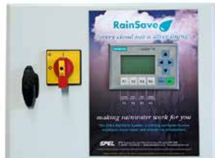
Controls incorporated into 'dry chamber' section of the storage tank
