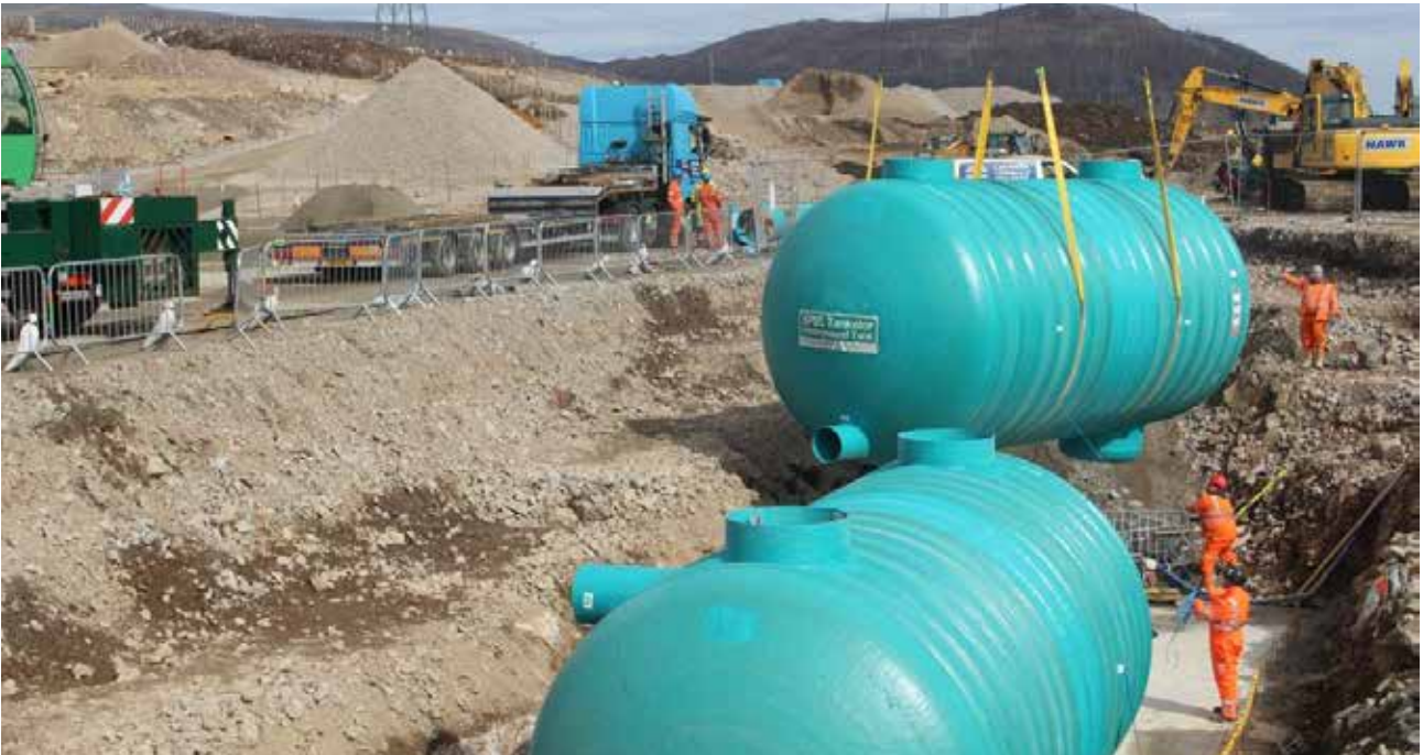
SPEL Tankstor® tanks. One with pump sump for the SPEL DrainGuard System
